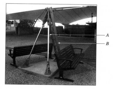
(i) A support for a public shaded area is shown in the photograph. Two types of members, A and B, are used to distribute the forces created by the weight of the fabric.
