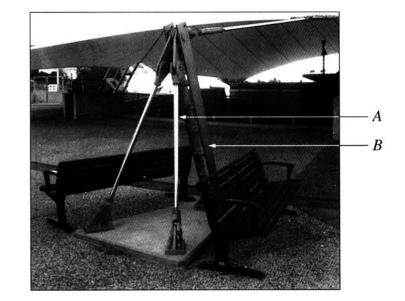
(i) A support for a public shaded area is shown in the photograph. Two types of members, A and B, are used to distribute the forces created by the weight of the fabric.
